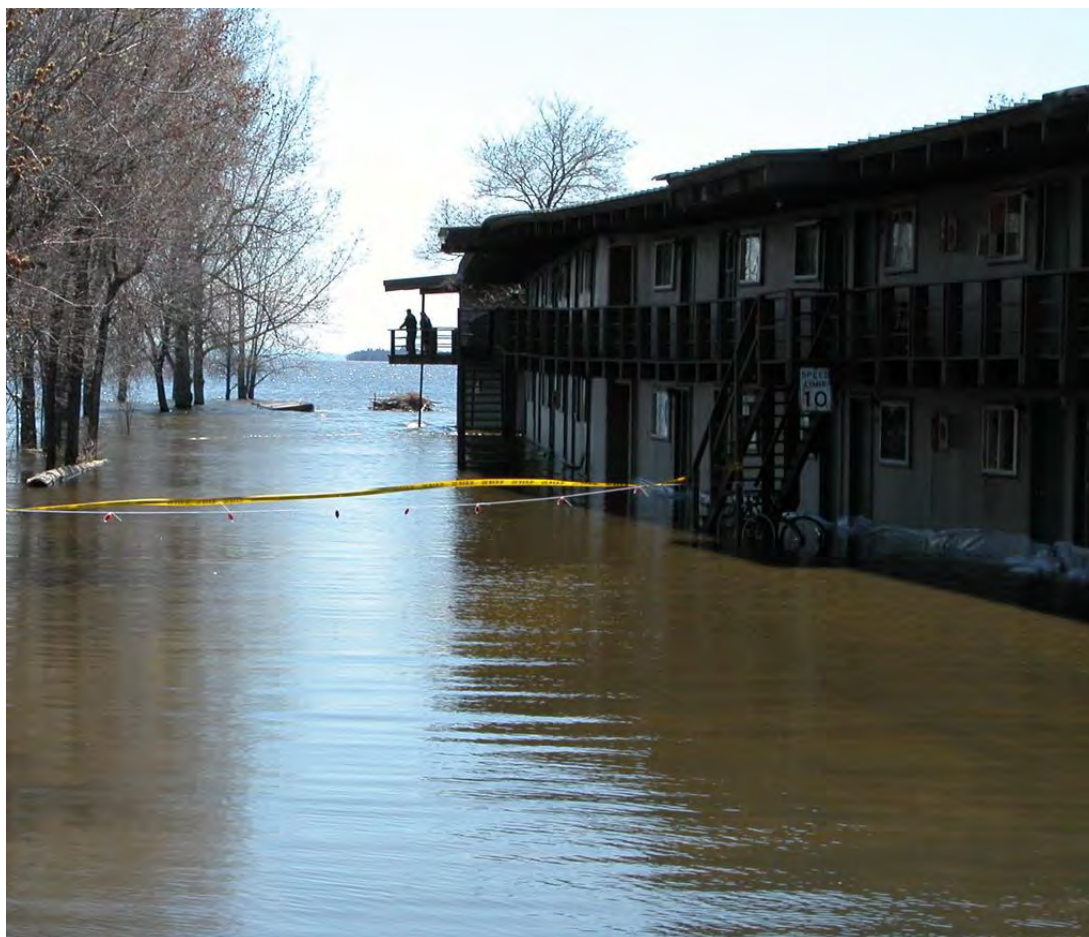
Photo shows the high level of the lake in 2011, the Lakeside Apartments buildings were inundated and later had to be demolished as a result of flood damages (image source: wamc.org)
